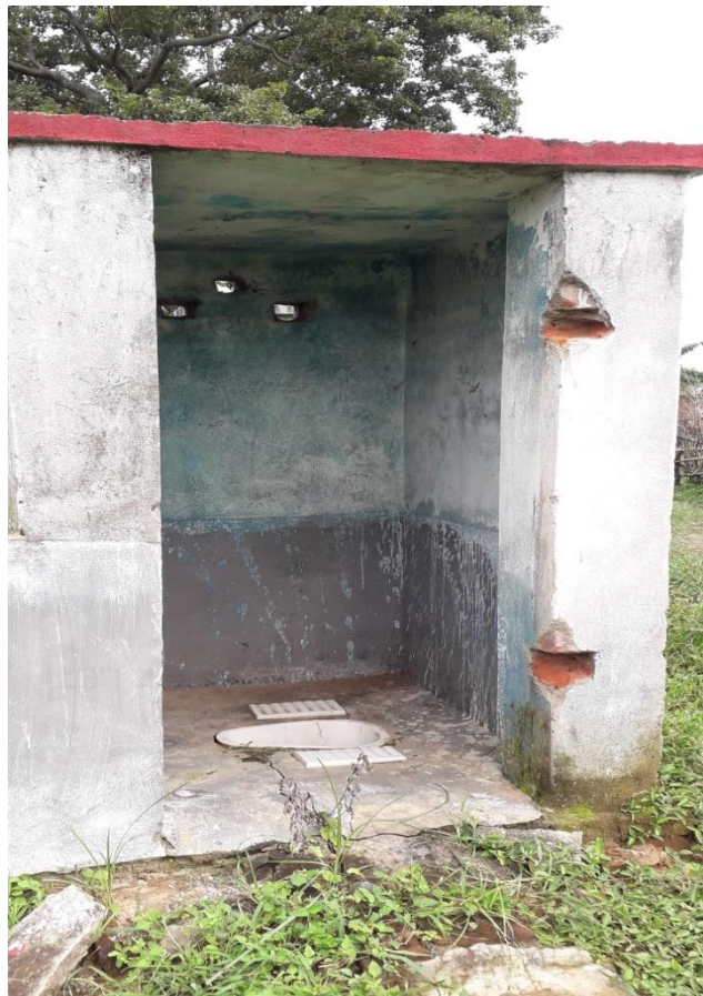
Toilet constructed under the SBM in Jharkhand – already without a door Photo Credits: Radhika Borde
